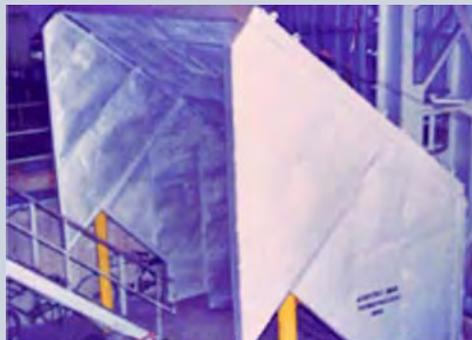
The Acoustic cladding material being assembled around the Blower casing
