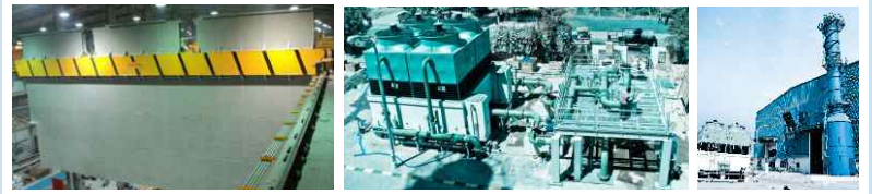
Multi - Disciplinary Turnkey Engineering Projects
